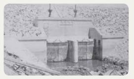
Floodgate Construction of Myoungji Dam (Myeongji-myeon, Gimhae-gun) - Width 1.85 m, Height 1.25 m, Length 24.5 m - Cost 12,000 ¥ - Initiation 1935/11/01. Completion 1936/03/31.
